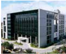
Taoyuan Technology Center (Green Building)
